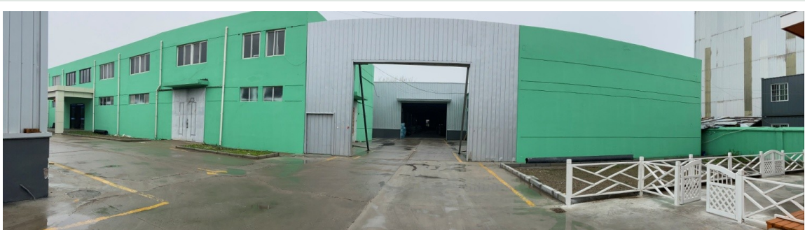
Factory Yard & Logistics Access Open yard space for production and material movement
